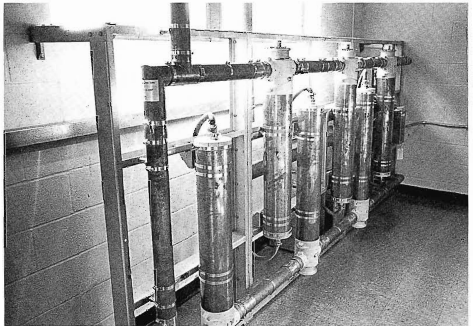
Wall-mounted Vistigial Sideband Filter for TT-50FL.
