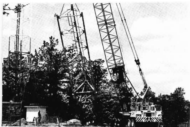
Crane hoists first section of 2,000 ft. WRAL tower into position.
