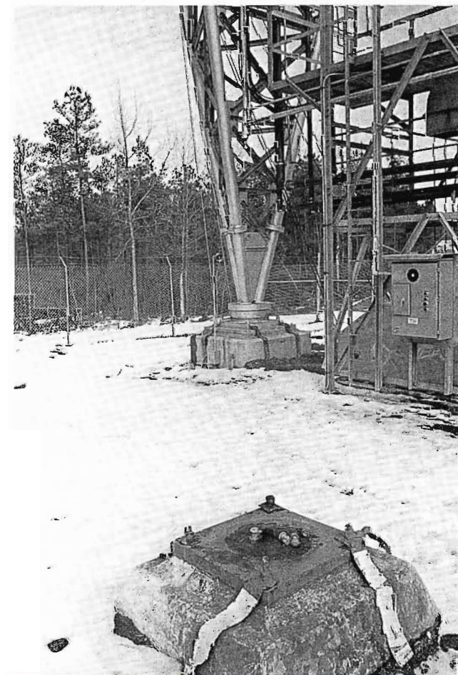
Base of dismantled old tower in foreground. New tower was erected within 30 feet of the existing tower.
