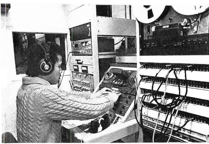
Audio control—8-track audio system provides separate sound and can be interlocked with SMPTE time code to AE-600 tape editing system.
